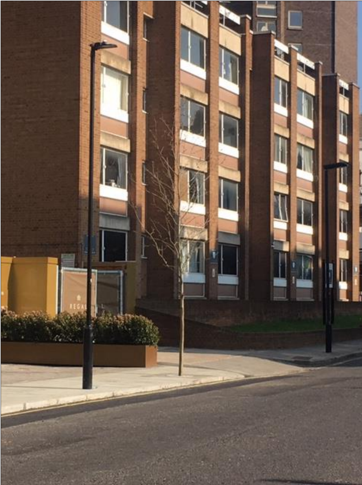
Existing Lodge Road elevation
